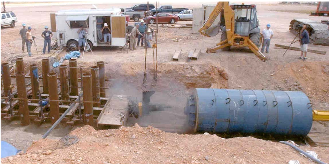
Figure 1.1: Lateral Static testing (S.R. Johnson, 2003a).
