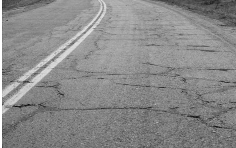
FIGURE 2.4 Block cracking.
