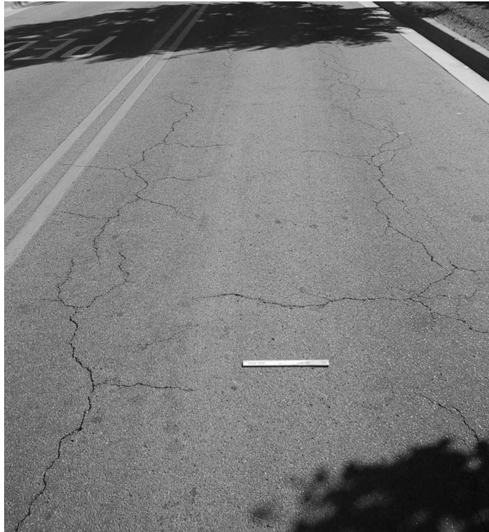
FIGURE 2.1 Longitudinal cracking.
