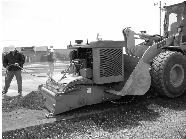
FIGURE 2.6 Portable asphalt recycling machine.
