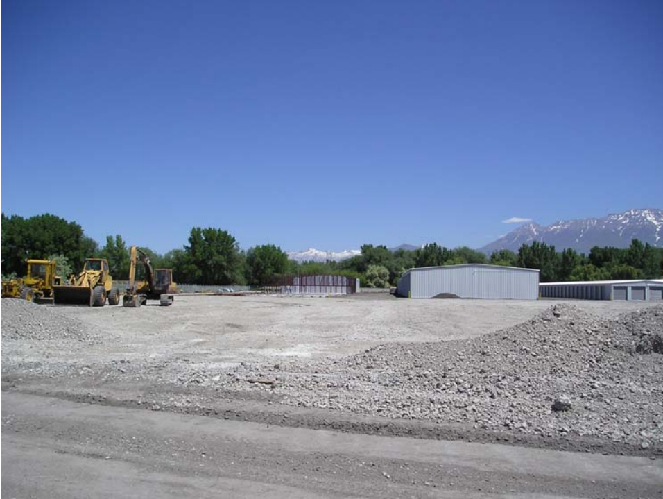
FIGURE 4-1 Unpaved recycled concrete material field site.
