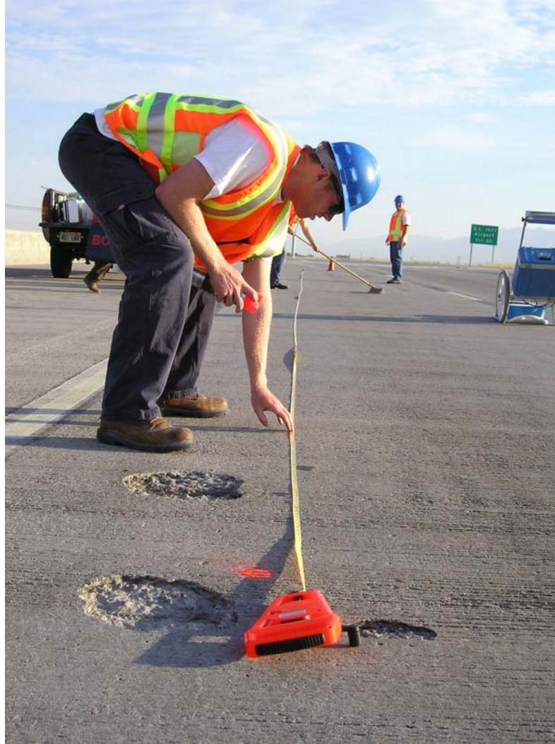
FIGURE 3.2 Stationing the test area.
