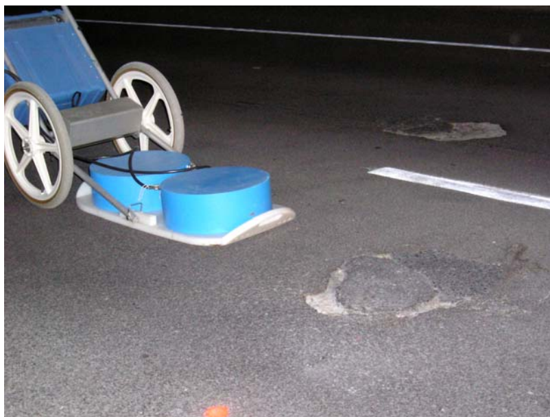
FIGURE 4.43 Concrete distresses exposed through overlay on bridge C-637.
