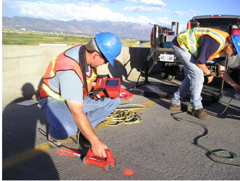
FIGURE 3.12 Locating the steel reinforcement.
