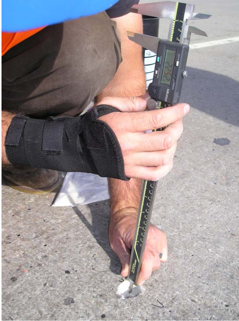
FIGURE 3.14 Measuring the depth of steel reinforcement.
