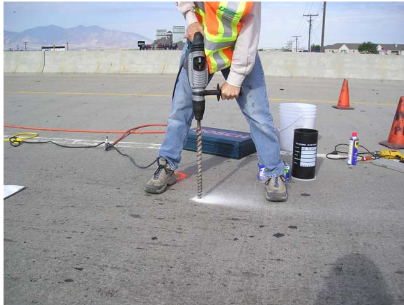
FIGURE 3.13 Drilling to expose the steel reinforcement.
