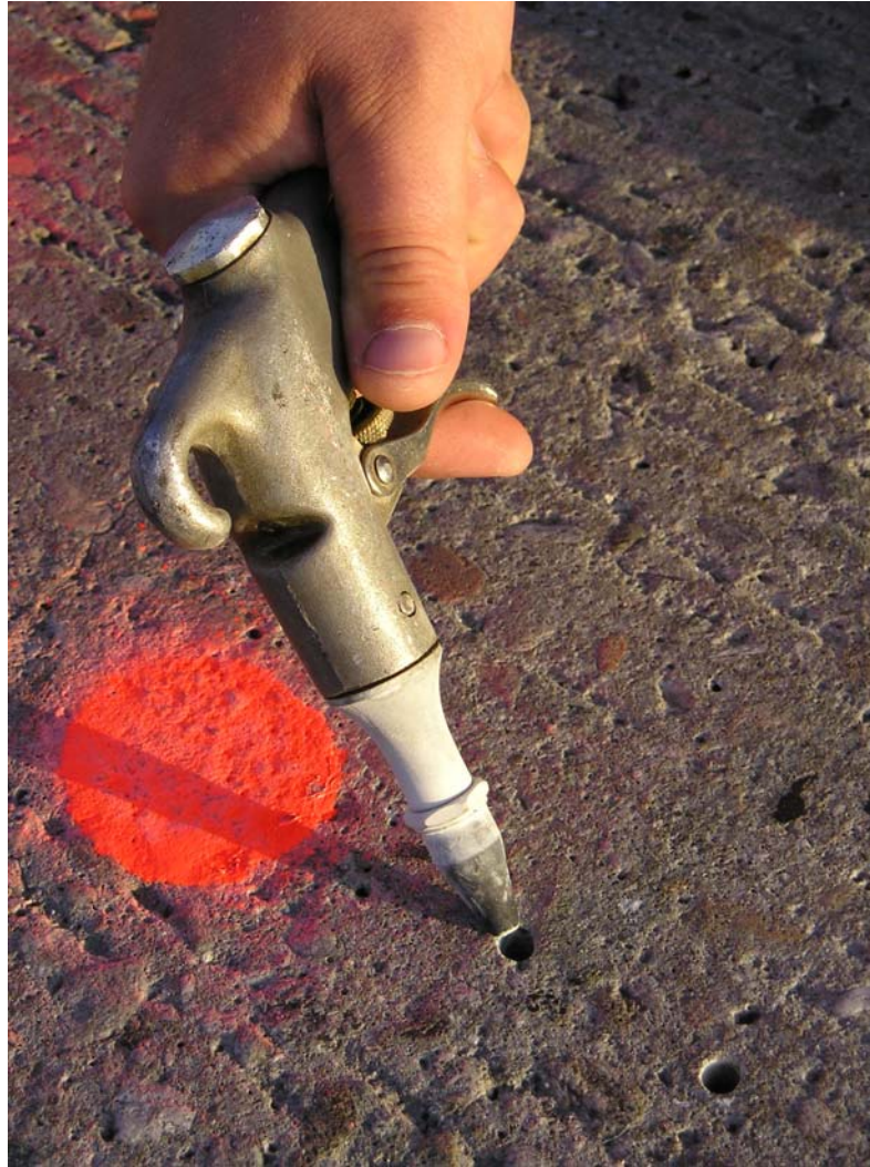
FIGURE 3.9 Cleaning test holes with compressed air.
