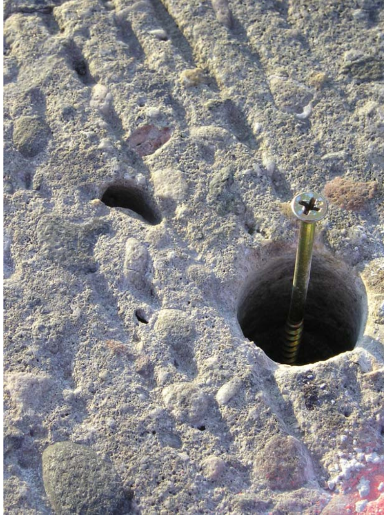
FIGURE 3.15 Screw installed in steel reinforcement.
