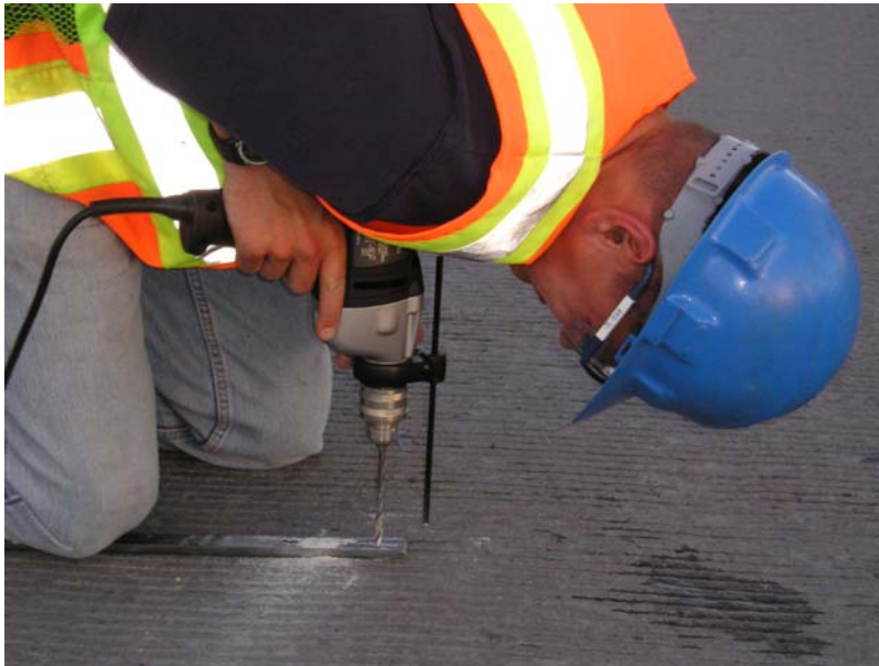
FIGURE 3.8 Drilling holes in preparation for resistivity measurements.
