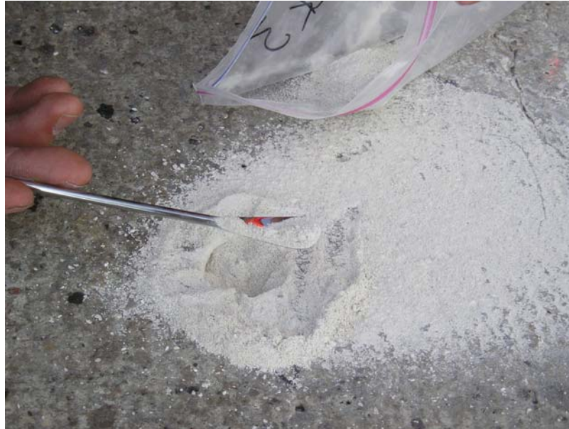
FIGURE 3.20 Collecting pulverized concrete for chloride concentration analysis.
