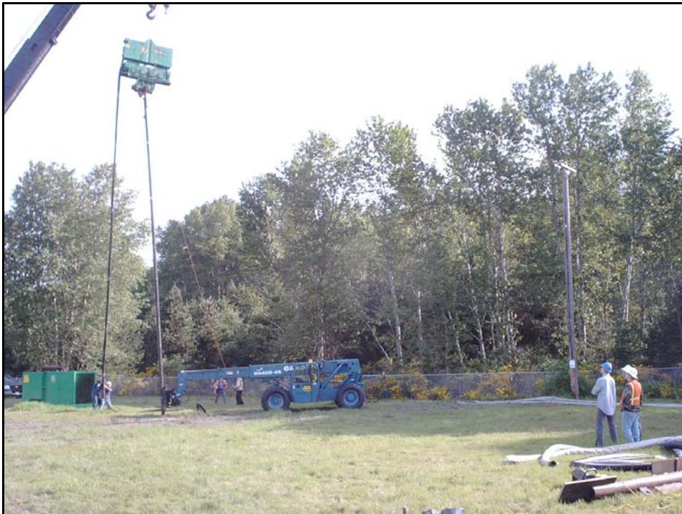
Figure 9-9 Installation of Blast-Holes by Vibro-Hammer
