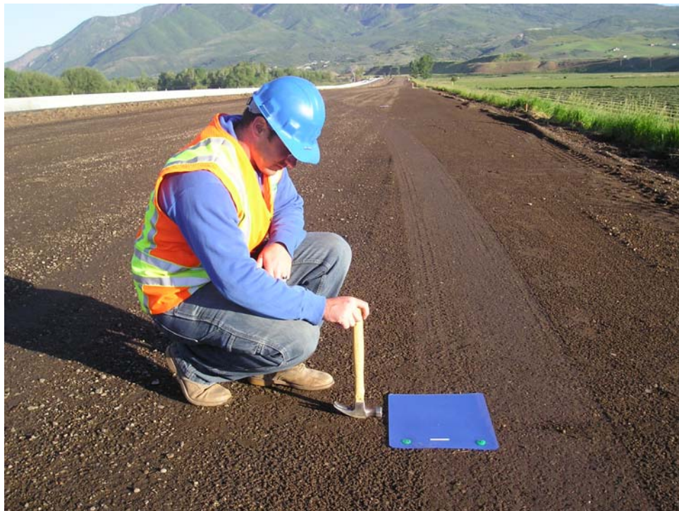
FIGURE 3.5 Placing cement collection sheet.
