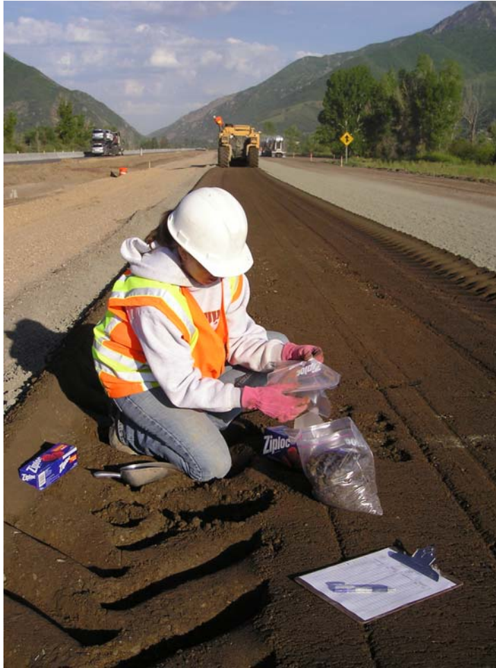
FIGURE 3.8 Sampling base material after cement mixing.
