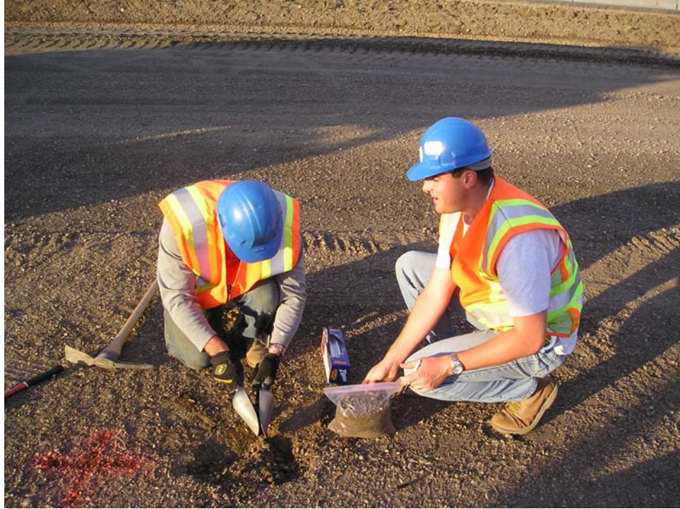
FIGURE 3.4 Sampling base material before cement placement.
