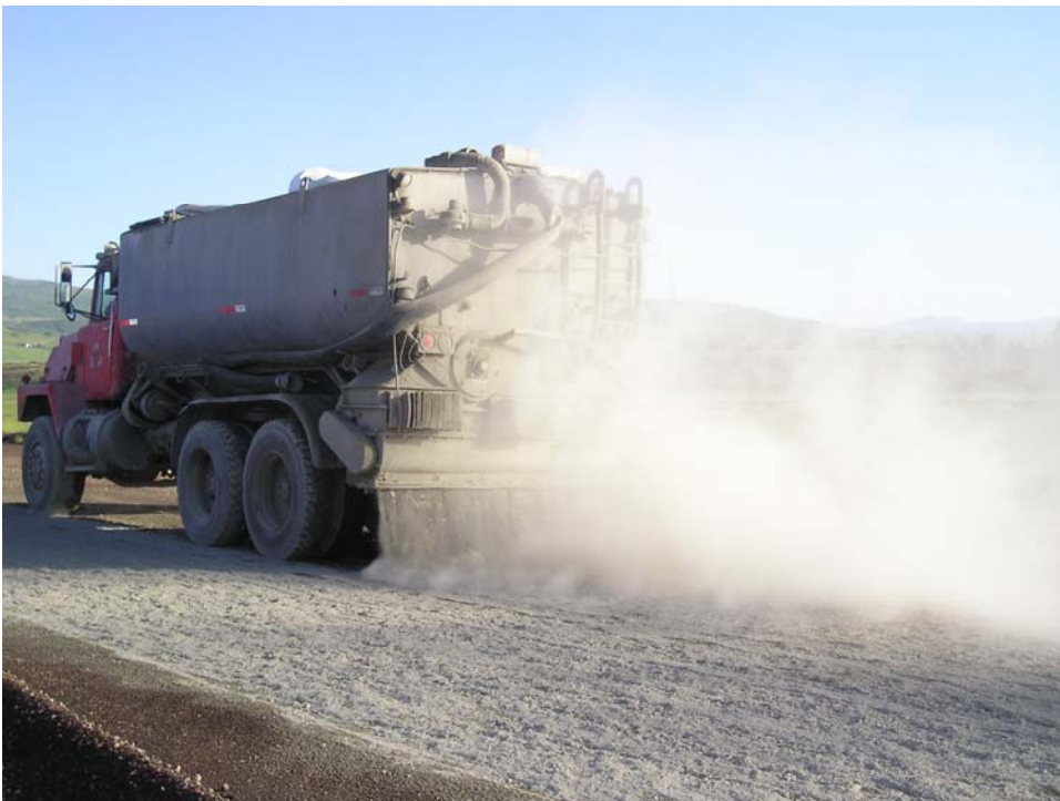
FIGURE 2.2 Cement placement process.
