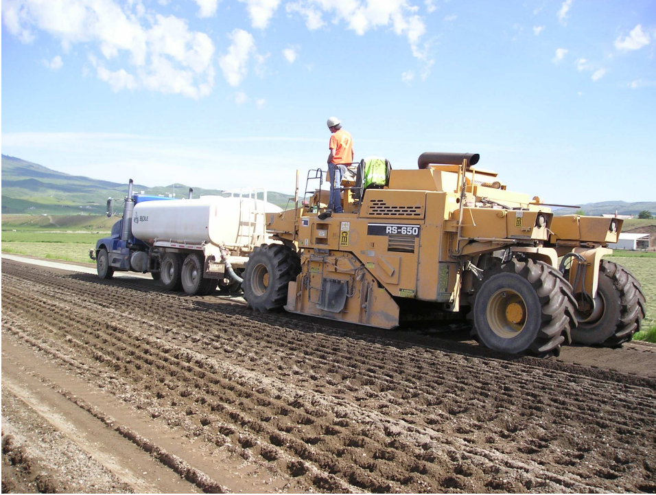
FIGURE 2.1 Reclaimer mixing cement-treated base material.
