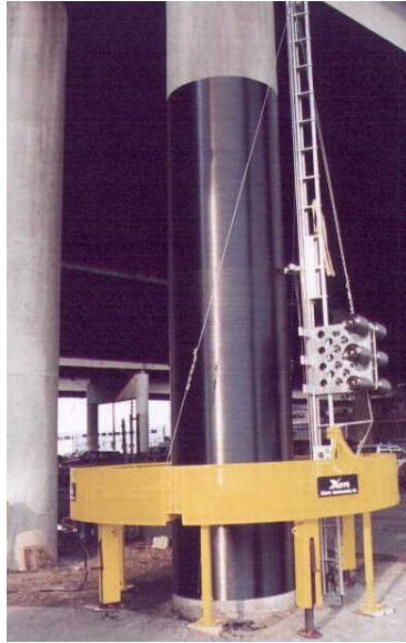
Figure 1.3 The ROBO-Wrapper I™. A freeway column retrofit filament winder (XXsys, 2004).
