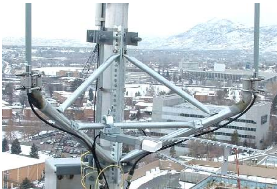
Figure 3-3 Close-up of antenna mounting bracket for two omnidirectionals and vagi
