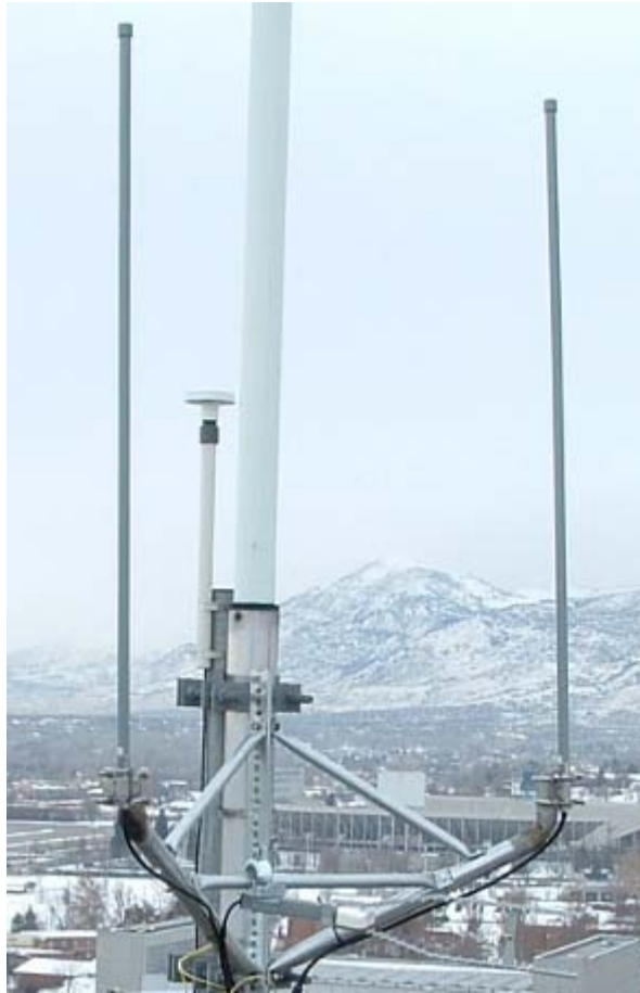
Figure 3-4 Full antenna mounting assembly on Kimball tower
