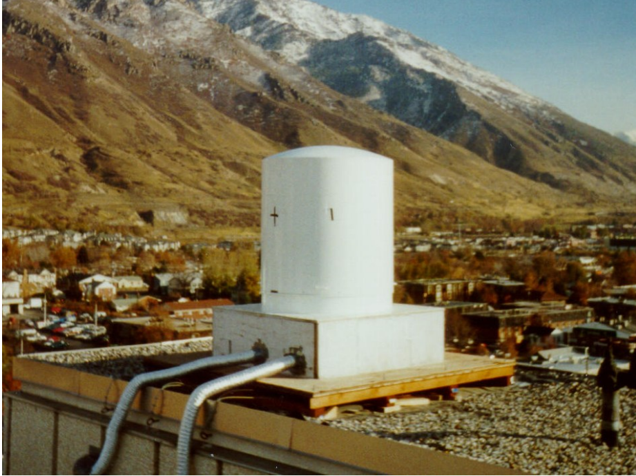
Figure 2.2: Receiver of the SeaWinds Calibration Ground Station at BYU, Provo, Utah. Ducting tubes pump cool air into the radome and protect sensitive cables connected to computers below.
