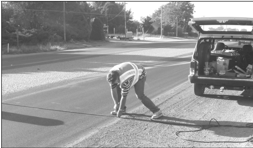
Figure 4. Placing the Speed Tubes
